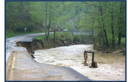
Vulnerability of infrastructure is another important consideration.
