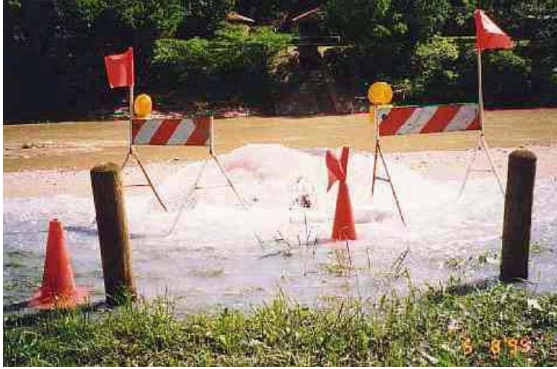
Figure 9-5. Combined sewer overflow near a stream. Source: USEPA, 2007.
