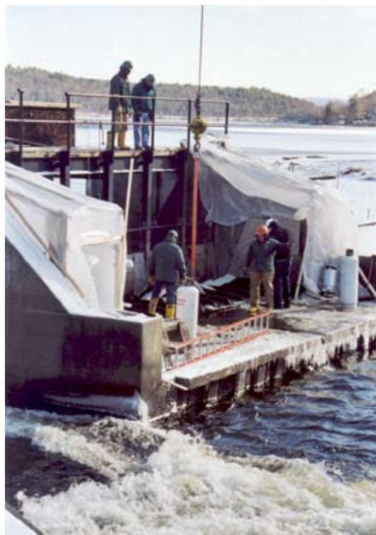
Figure 1-6. Installation of the automated spillway gates is an example of an upgrade at the Mascoma Lake Dam on the Mascoma River in Lebanon. Source: NH-DES Dam Bureau.
