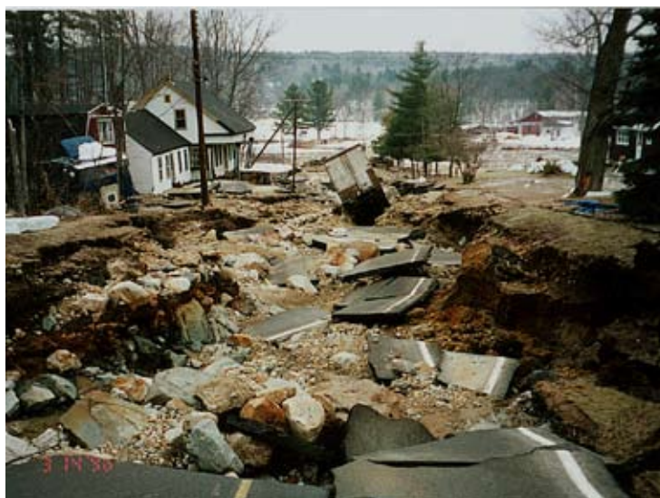
Figure 11-3. Meadow Pond Dam in Alton looking downstream at road damage. One life was lost when the dam failed. Source: NHDES, Dam Bureau File Photo.
